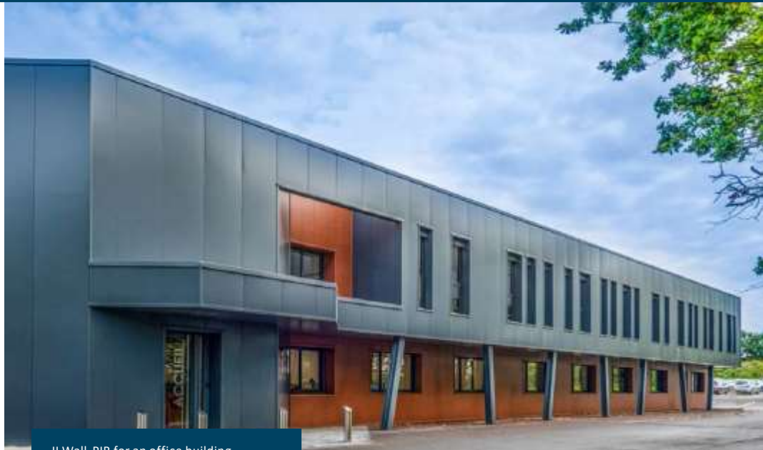
Jl Wall PIR for an office building.
