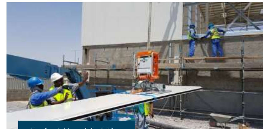
Use of sandwich panels for cladding.
